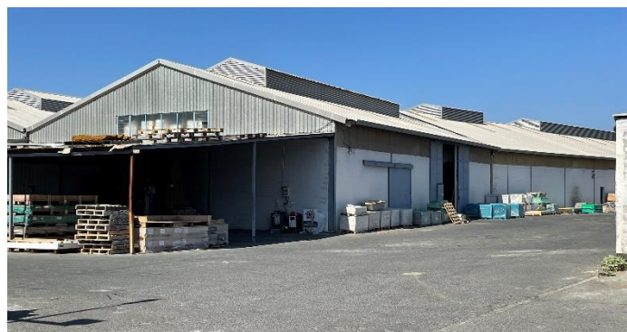
Figure 2 EKA Group's main warehouse
